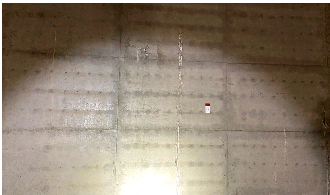
Same point on wall 7 weeks later – cracks fully healed with no water leakage against constant hydrostatic pressure.
